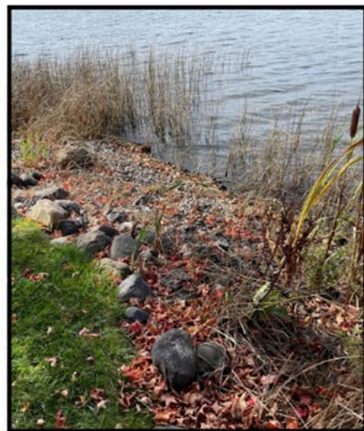
The larger boulders on this shoreline are where the waterline stays most of the time. This year the water was at least a foot below normal.
